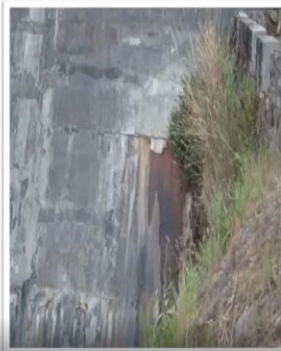
downstream face of Khandong Dam
