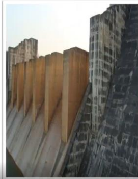
Khandong Dam – Spillway view
